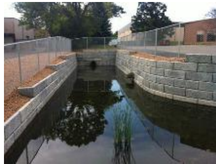
Figure 3-11 Gravity Wall Retention Pond, Plymouth, MN (ReCon Retaining Walls, n.d.)
