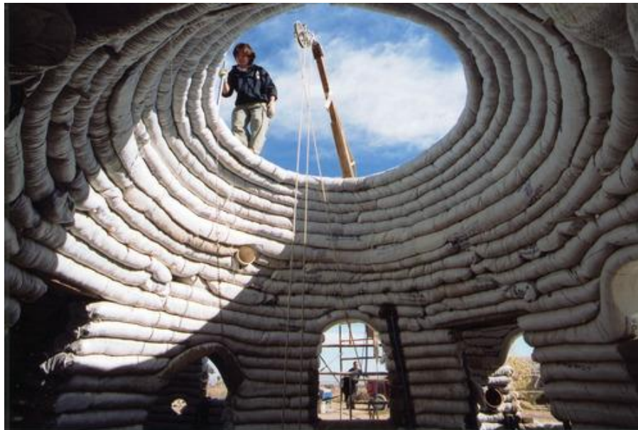
Figure 3-14 SuperAdobe structure in construction (CalEarth n.d.)
