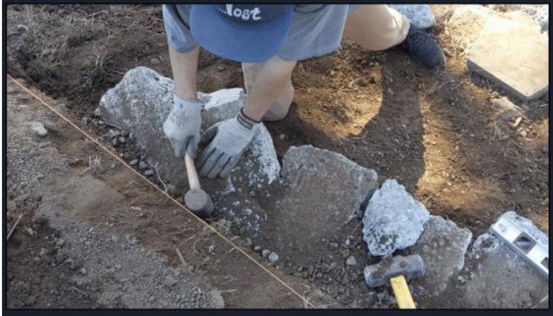
Figure 5-11 Massaging gravel and soil backfill into place
