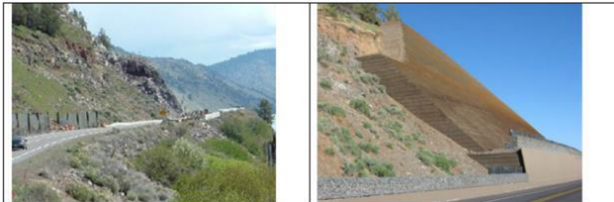
Figure 3-10 Before/after of US 97: Modoc Point - Hagelstein Park Project (Hilfiker Retaining Walls 2015)
