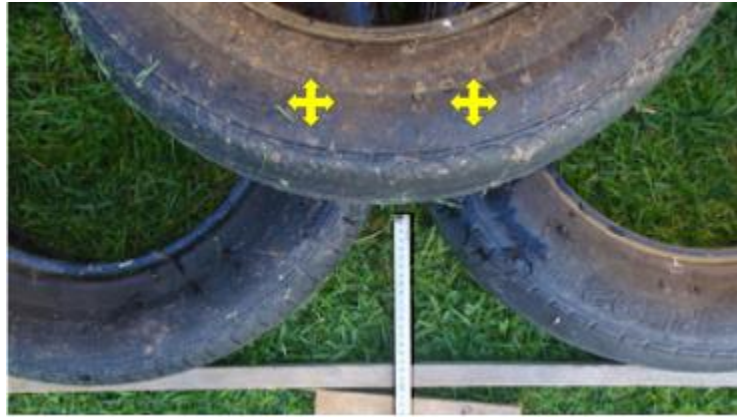
Figure 5-10 Placement of second row of tires.
