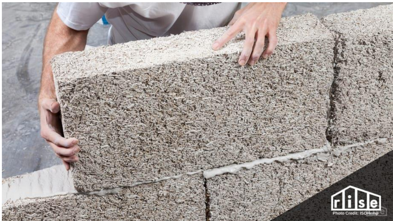
Figure 2-7: Hempcrete bricks being placed down to raise a wall (Rise)
