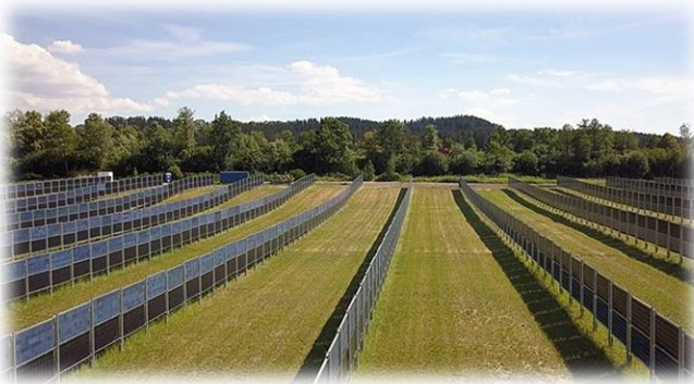
Between-the-row agrivoltaics
